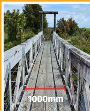
Mahinapua Creek bridge
